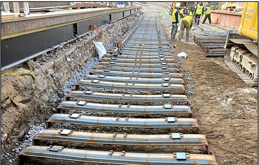
Rail installation on formed steel ties on the Manitou And Pike's Peak Railway. – Photo from M. Garfalo.
